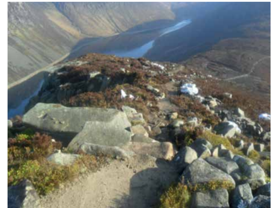
Upland Path Works on Binnian Mountain
